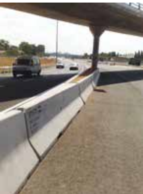
Highway no. 5. Double restraint system. Model: DB80AS/6M Double Row
