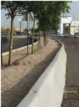
Highway no. 75 Haifa Bay Combination of greenery and an avenue of trees in a double restraint system. Model: DB80AS/6M Double Row
